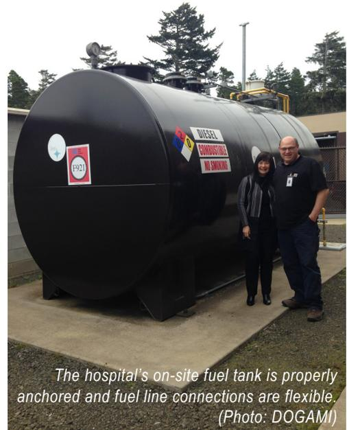
The hospital's on-site fuel tank is properly anchored and fuel line connections are flexible. (Photo: DOGAMI)
